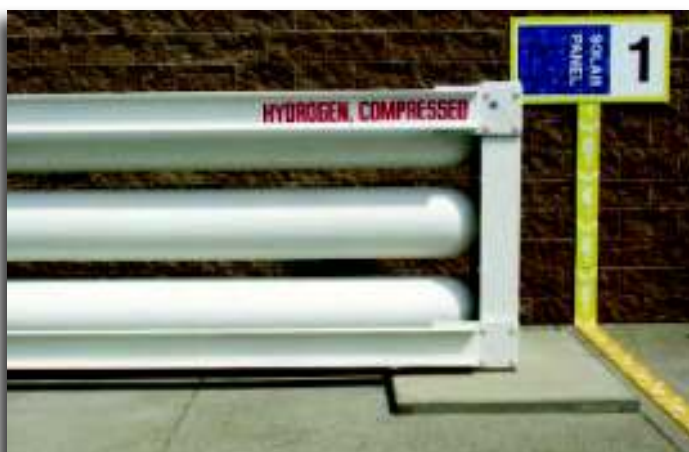
Compressed hydrogen storage tanks at the SMUD solar-powered hydrogen vehicle fueling station in Sacramento, California.
